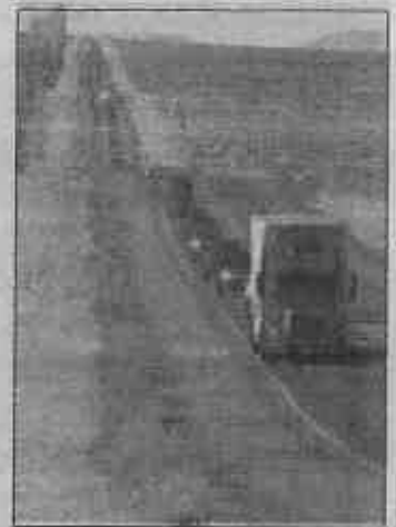
Construction could begin as early as late 2018 on the roughly $60 million widening of a 5.6-mile stretch of Highway 395. (JAMES OUIGG, DAILY PRESS)
